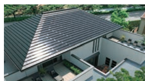
Sekisui House proprietary tile-based solar power generation system
